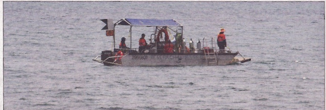
AURECON: Aurecon workers were seen conducting measurement exercises near the Perry Harvey Jetty on Friday.
