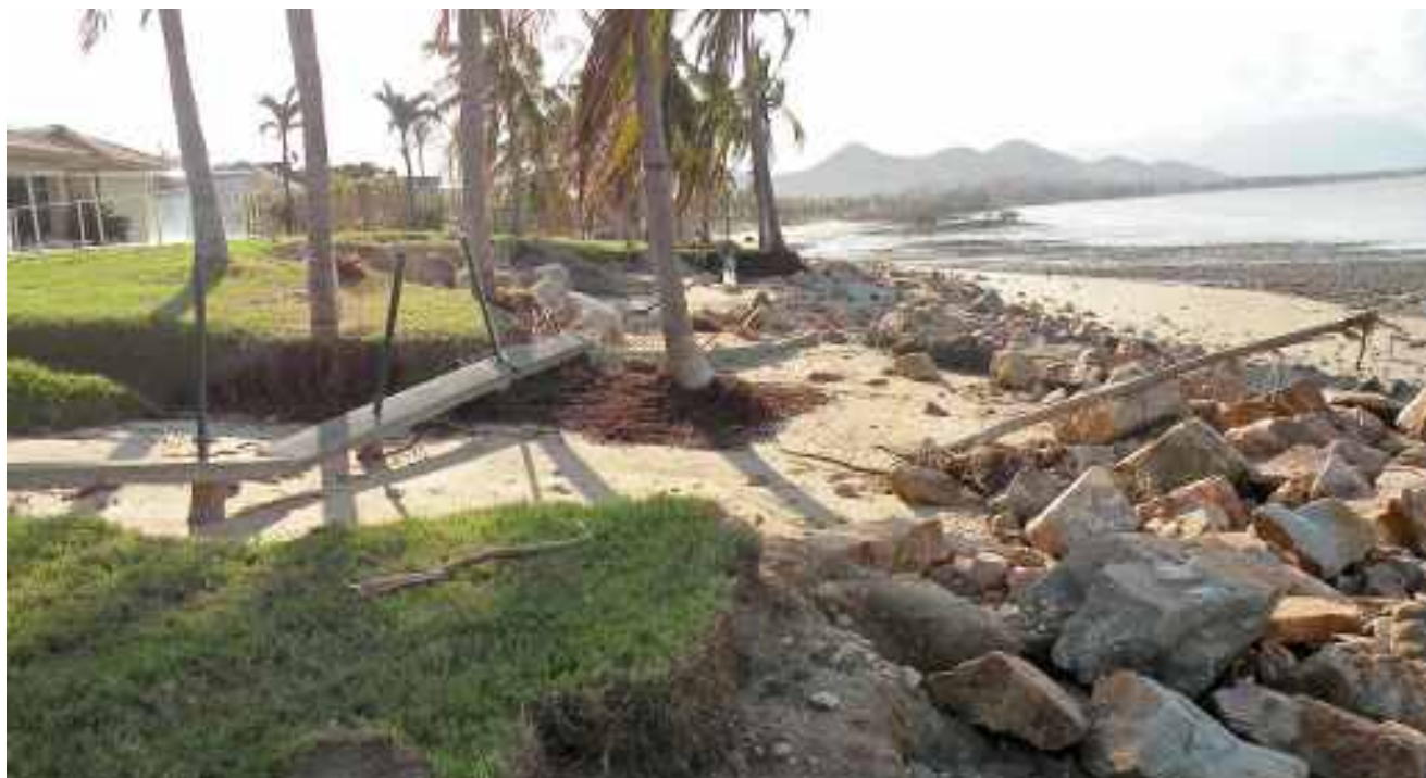
"Port Hinchinbrook" a month after cyclone Yasi, towards low tide. Foreground: rock retaining walls and the seafront back yards of the housing estate scattered across the foreshore, along with steel fencing and concrete footings.
