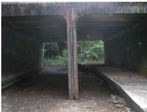
PLATE 1 – QDMR's large culvert trial. Note the raised platform allowing dry passage
