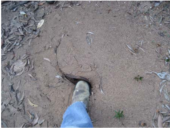
PLATE 16 – Wetpour safety surface having lifted from the culvert floor washed away and covered with silt (photographed late 2007).
